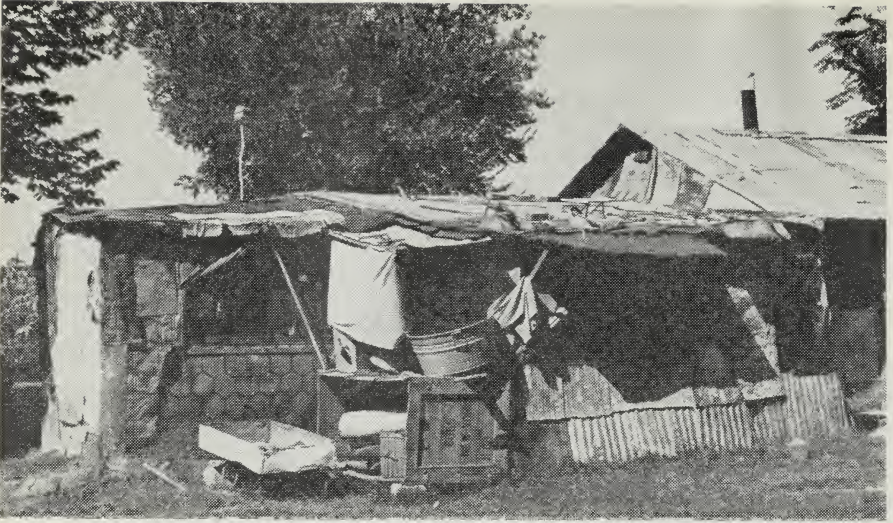
Shack and tent dwellings in Elm Grove camp inhabited by destitute families.
